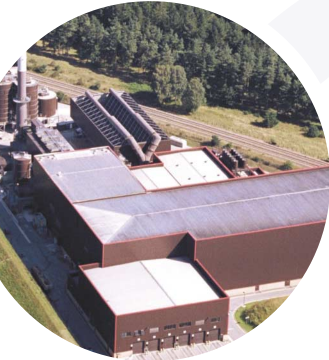
The world's third poultry-fired power station and Europe's largest biomass-fuelled electricity generator is located in the region
